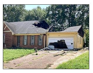
It has been determined that the residence **did have** a working smoke alarm. The structure sustained smoke, fire and water damage. Total damage is estimated at \$100,000.00 structure and \$20,000.00 contents. The origin and cause of the fire was determined to be an A/C unit that malfunctioned in the attic.
