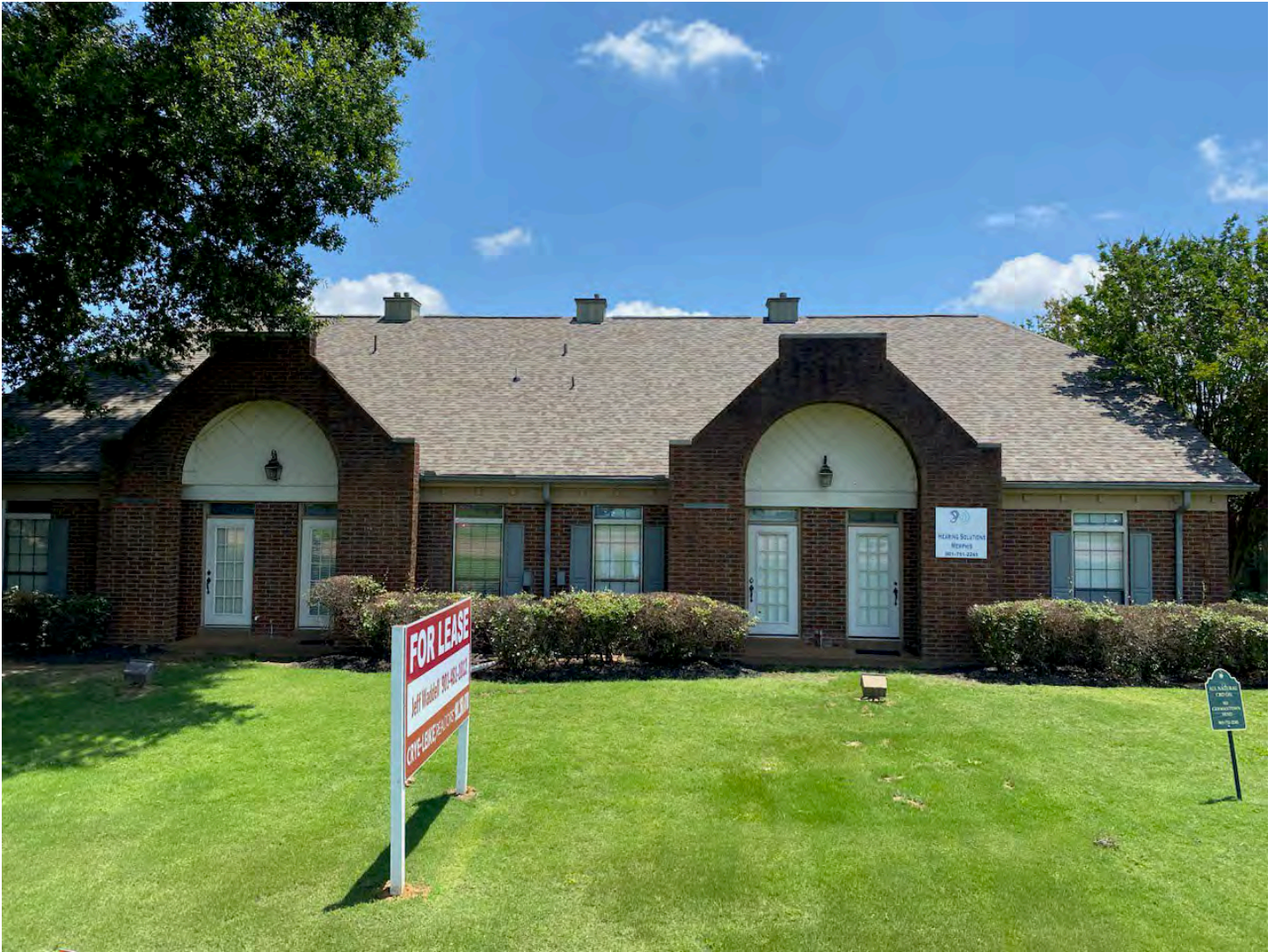
View of structure from Germantown Pkwy.
