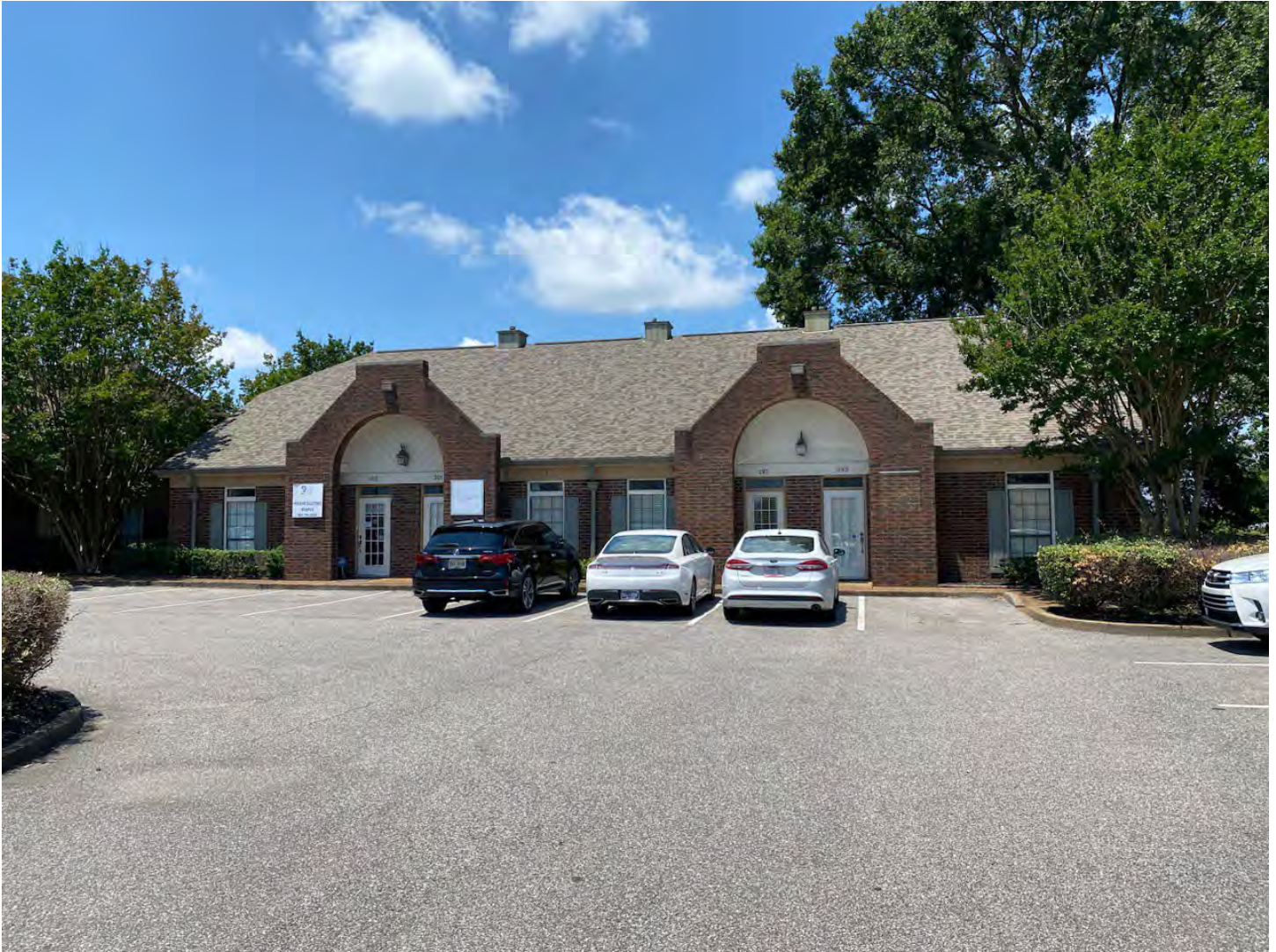
View of structure from Germantown Bend Cv.
