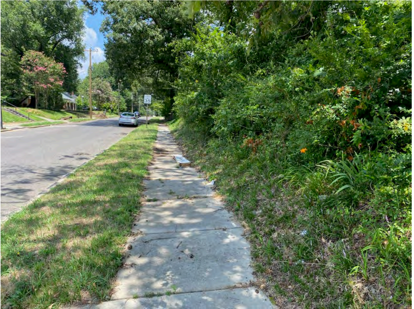
View north down Haynes
