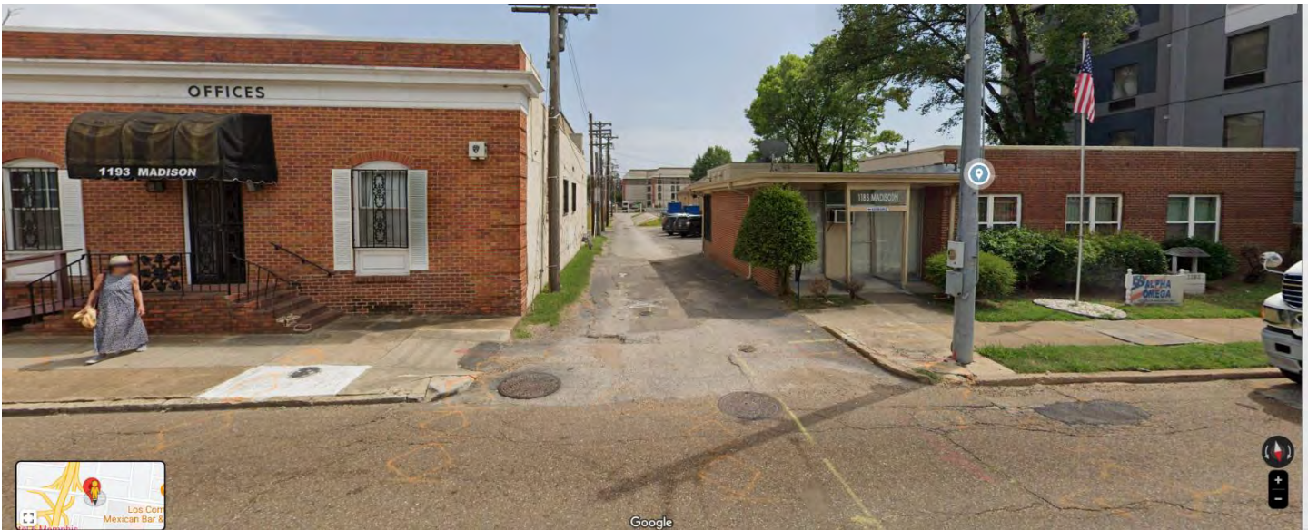
View of access point from Madison Avenue looking south
