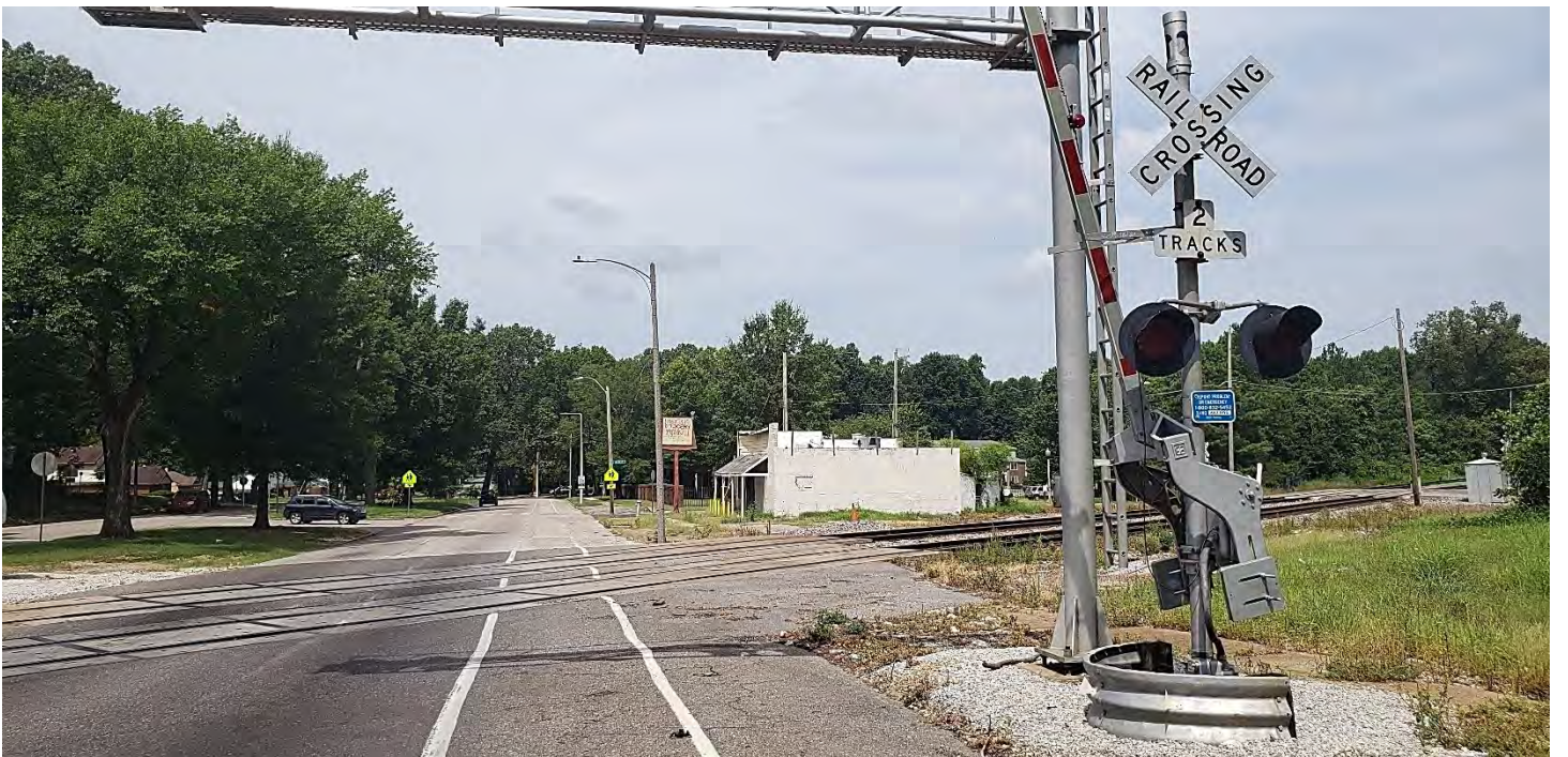
View of S Parkway E looking west
