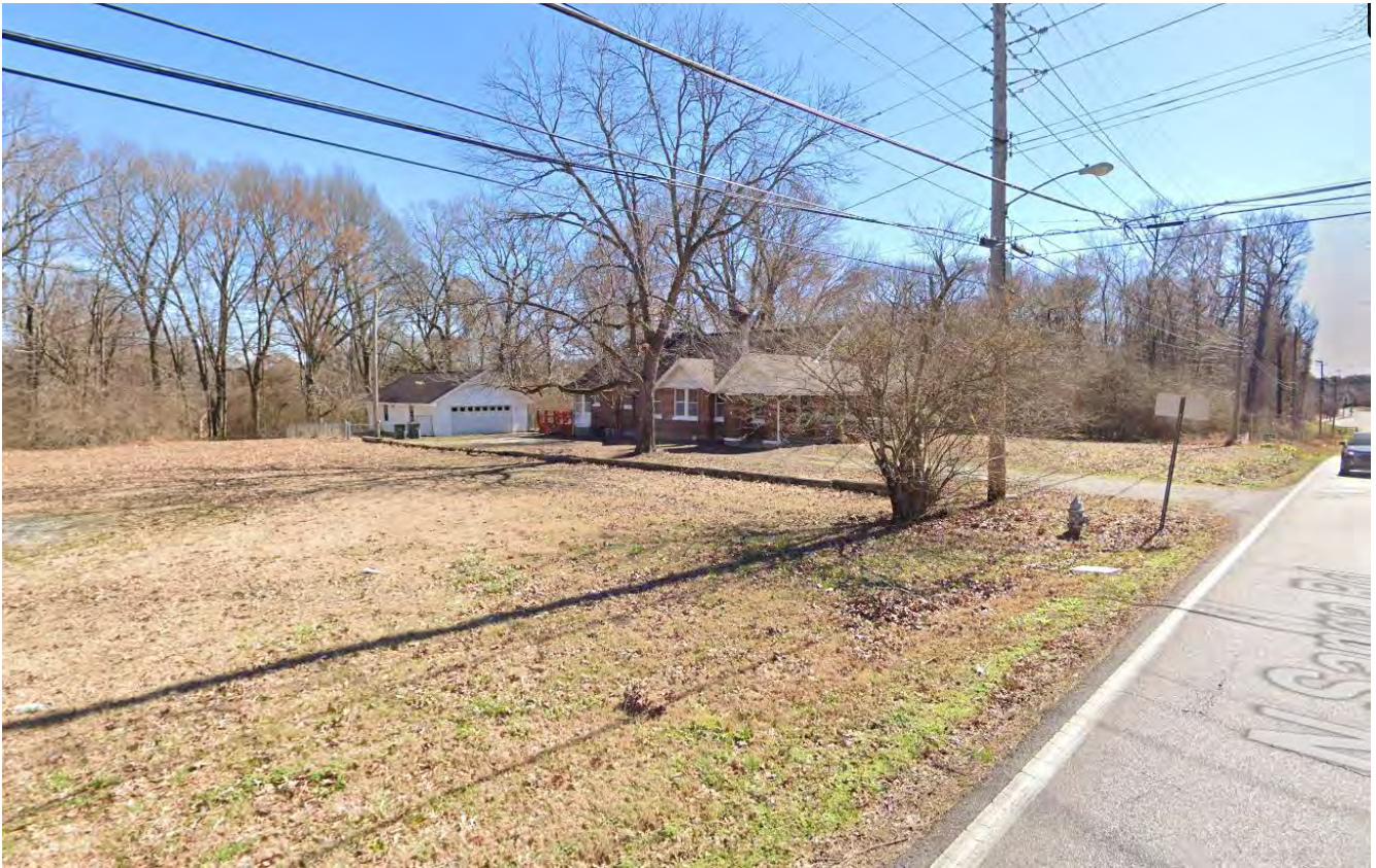
View of existing house to remain from New Sanga Road, Feb. 2023
