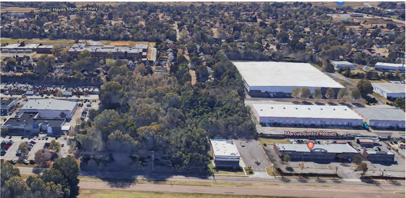
View of the subject property from US Highway 64
