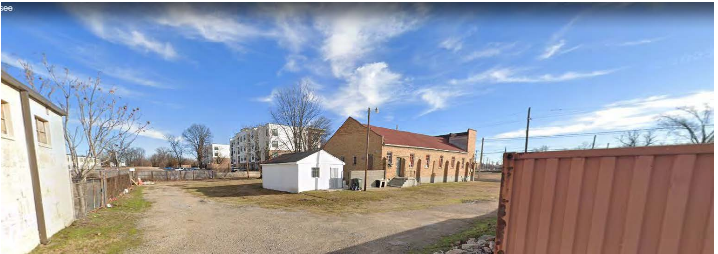
View of access point to the subject right-of-way from the ally (East)
