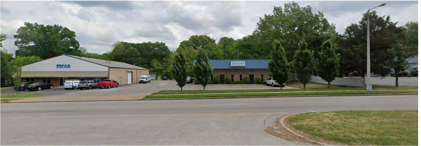
View of the subject property Sycamore View Road (Front)
