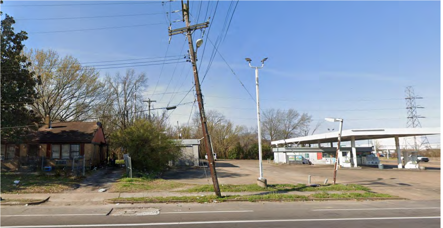
View of subject property from Macon Road
