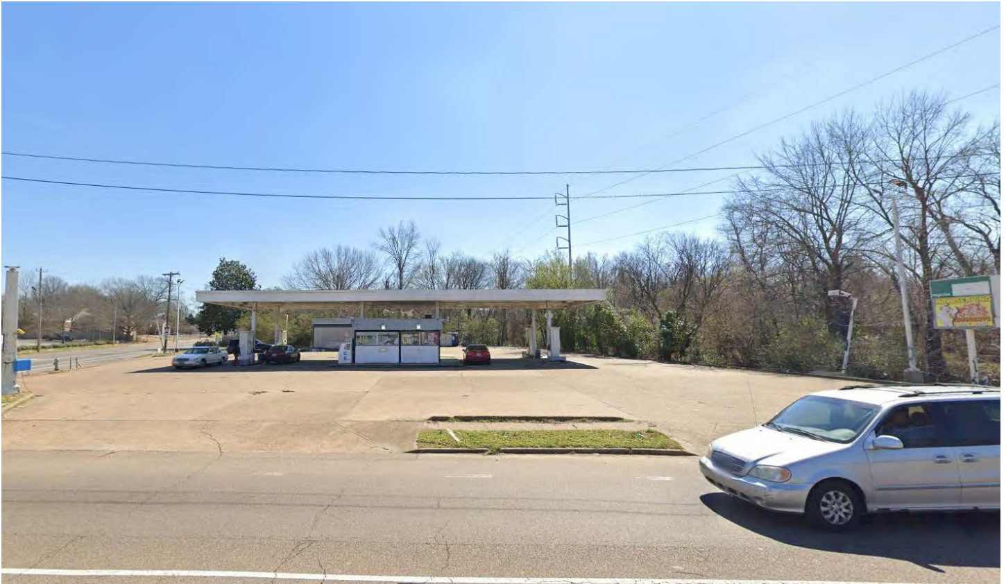
View of subject property from Jackson Avenue
