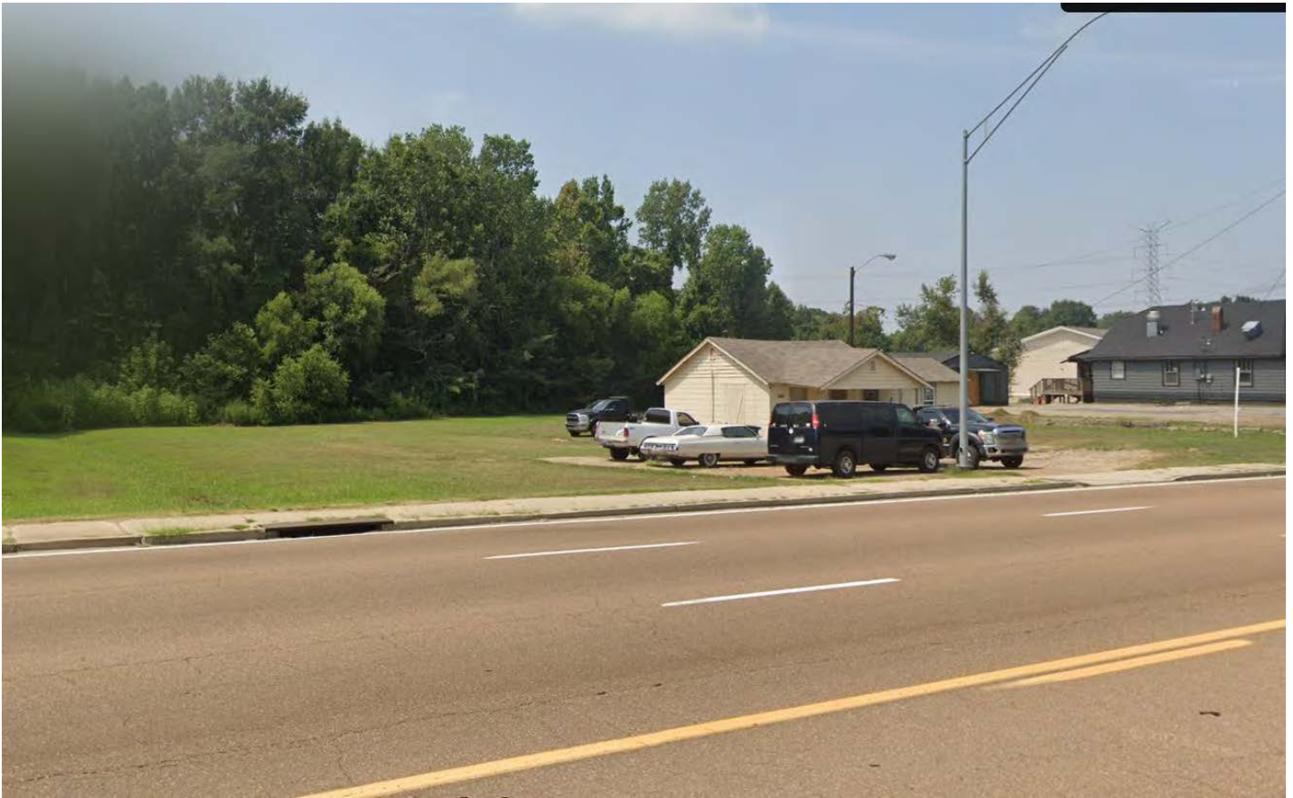
View of subject property looking north South Third Street
