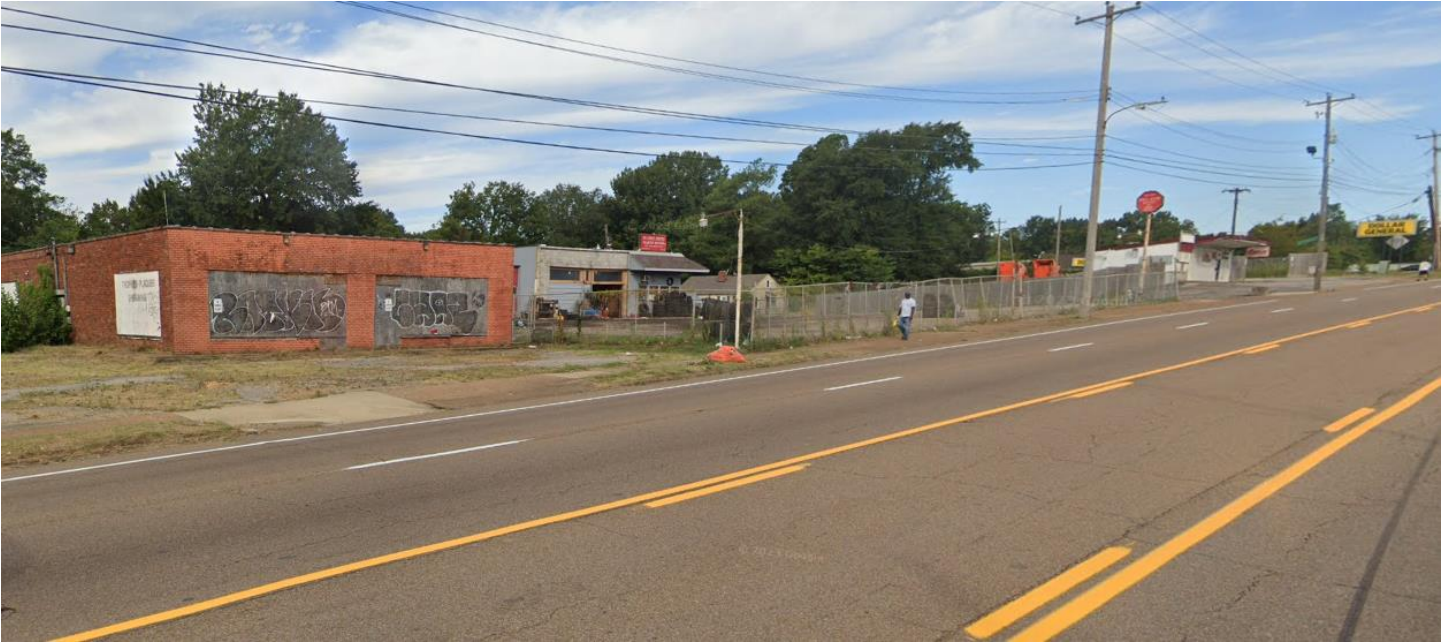
View of the subject property looking West on Lamar Avenue.
